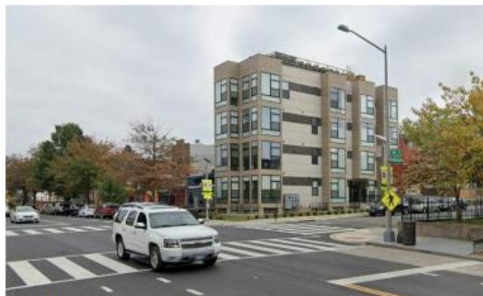
D. THE INTERSECTION OF 14TH AND RANDOLPH
